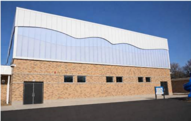
IPS Eliza Blaker Expansion , Meticulous Architects. Layered clouds incorporated into the facade as an energy and shading strategy ©Danpal
