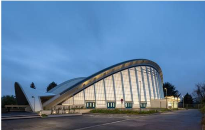
Grande Nef, Paris. Renovation preserved an iconic luminous profile while upgrading comfort, glare control and energy performance. Architect: Antoine Mercusot-Chatillon Architectes
