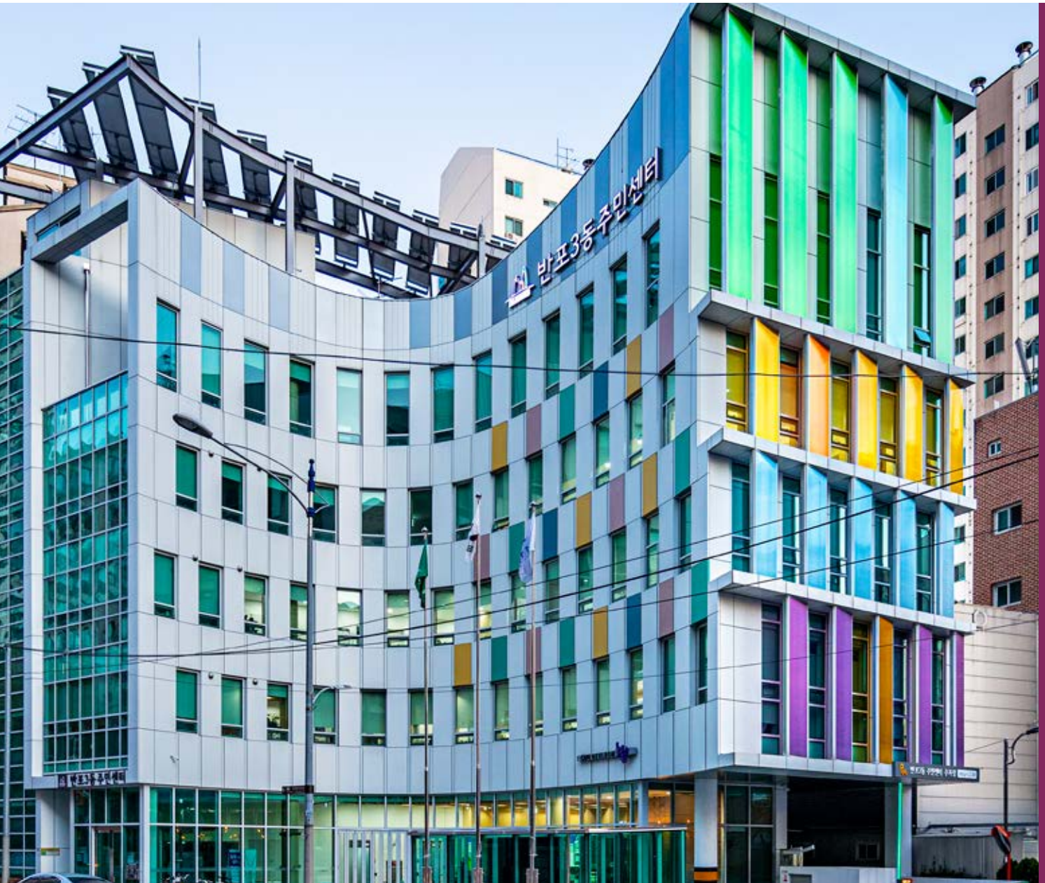
City Service Center, Banpo, 3 District in South Korea | Danpal® Louvre System
