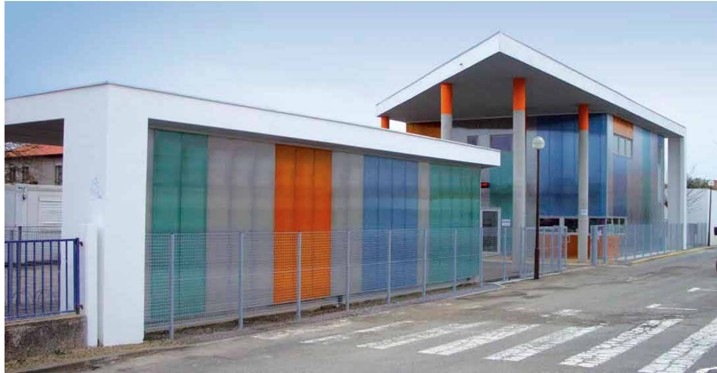
■ Fitting contractor: Miroiterie Lapegue, Dax (40) - Tel: 05 58 74 28 74 - Double Danpalon wall on a vertical aluminium frame: Danpalon 16600 sq. m. Green, Blue, Orange, Crystal.
