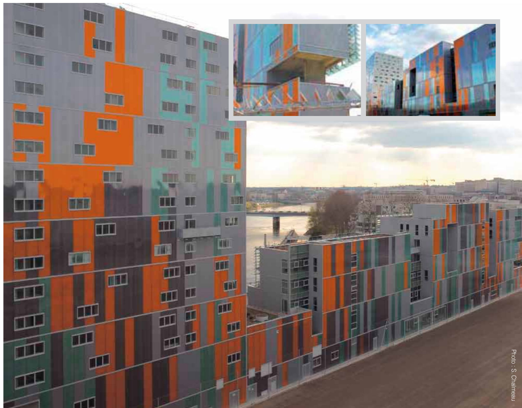
■ Fitting contractor: Cladding: Axima, Nantes (44) - Tel: 02 40 32 49 90 - Sunshades: Ateliers David, Guérande (44) - Tel: 02 40 24 90 34 Northside: 4400m 2 Danpalon 16 cladding, MC 1040 Aluminium, Green, Grey, Orange, Opal, Red - Southside (Sunshade): 2500m 2 Danpalon Blue, Crystal, Grey, Orange, Green.
