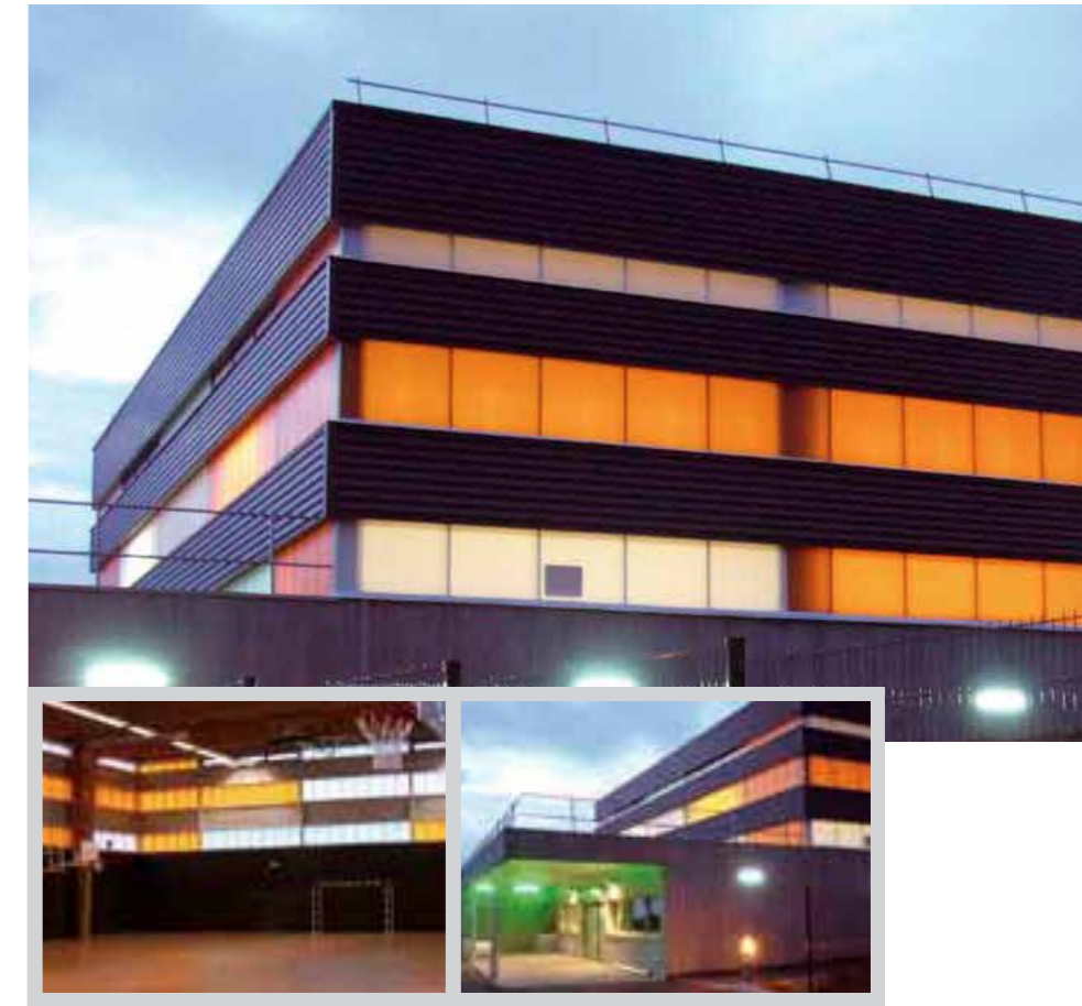
■ Fitting contractor: MARTIN G, Pont Evêque (38) - Tel: 04 74 16 17 77 - Danpalon Cladding 16 600 sq. m. Crystal Softlite and 1040 Crystal, 600 and 1040 Green Softlite and Orange.
