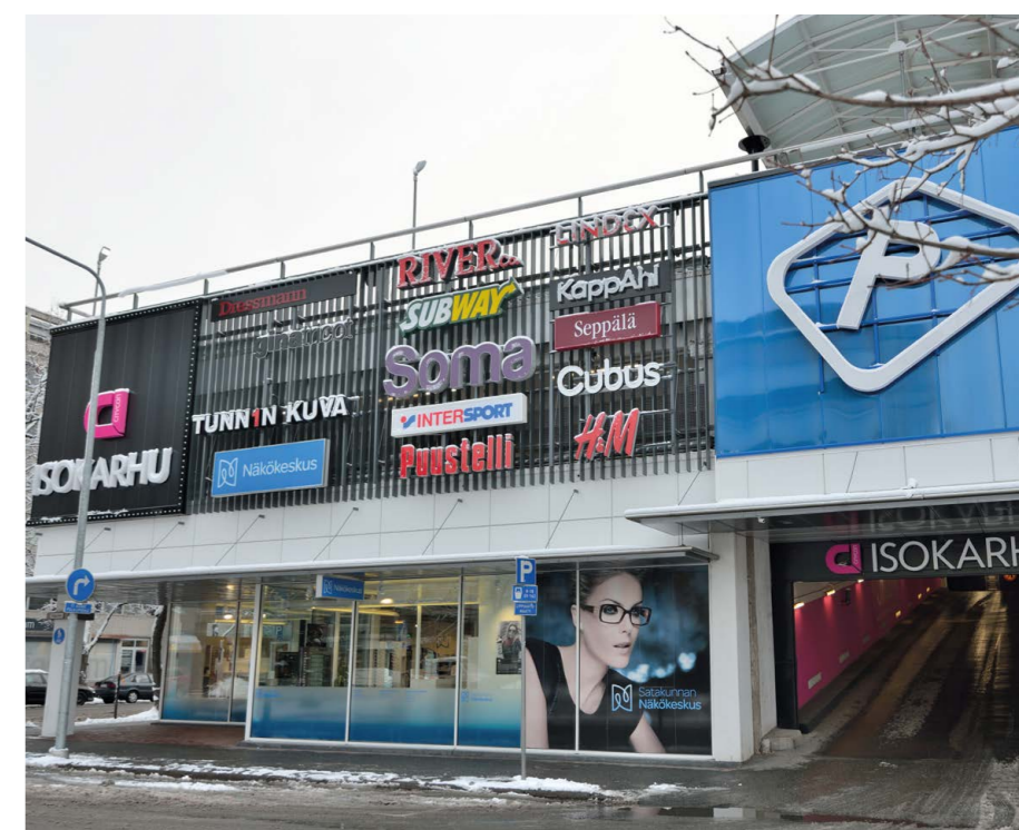
■ Ventilated Rainscreen, Danpalon® BRV 12, 900 mm, black Softlite, sapphire blue black eclipse Softlite, 220 m 2
