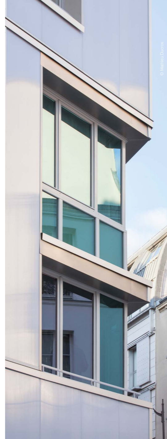
■ Ventilated Rainscreen, Danpalon® BRV 16, 1,040 mm, opal, 280 m 2
