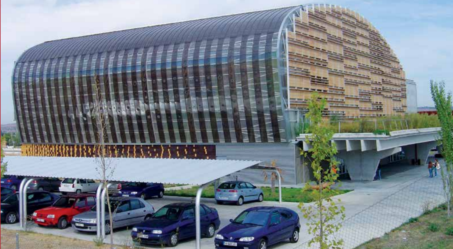
Office Building, Spain | Danpal® Compact | Architect: Pich Aguilera
